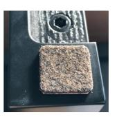
Glue on enclosed felt as base fort he spaker on the top plate.
